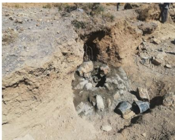
Figure 9. The operation of improving the aerator rod at the place of flood entering the Khumsian Qanat of Ashkazar.
