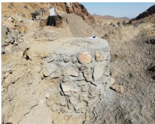
Figure 9. The operation of improving the aerator rod at the place of flood entering the Khumsian Qanat of Ashkazar.
